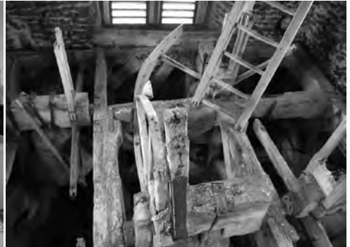
The old medieval framework before the bells were replaced.
