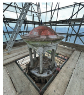
Stripped of lead - original cupola
