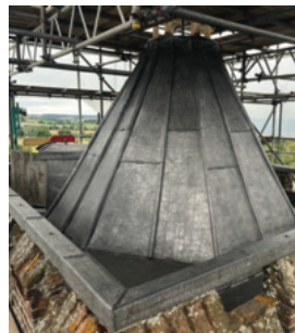
New modern materials now cover the spire & valley gutter
