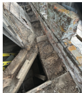
Lead removed showing the structure below
